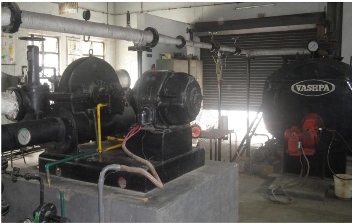
**Fig: Turbine Coupled to Generator**
