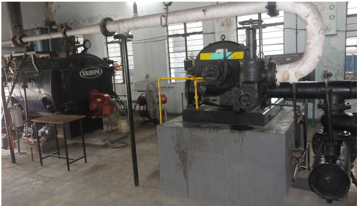
Fig: Boiler with impulse steam turbine
